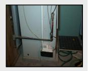
When selecting a new condensate pump it is important to have an accurate head measurement, GPM (gallons per minute), HP (horsepower), and voltage rating.
